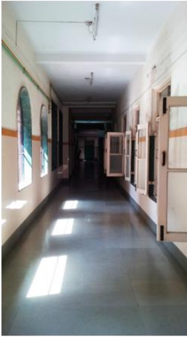
Corridors along wards on the western side, reducing the light intensity in the wards.
